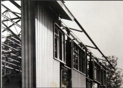
BSIF house under construction Image: Non-Standard House Construction
